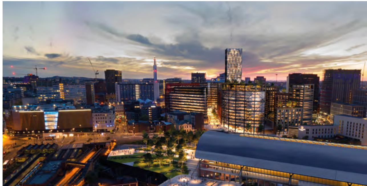
City Quarters at Martineau Galleries, Birmingham
